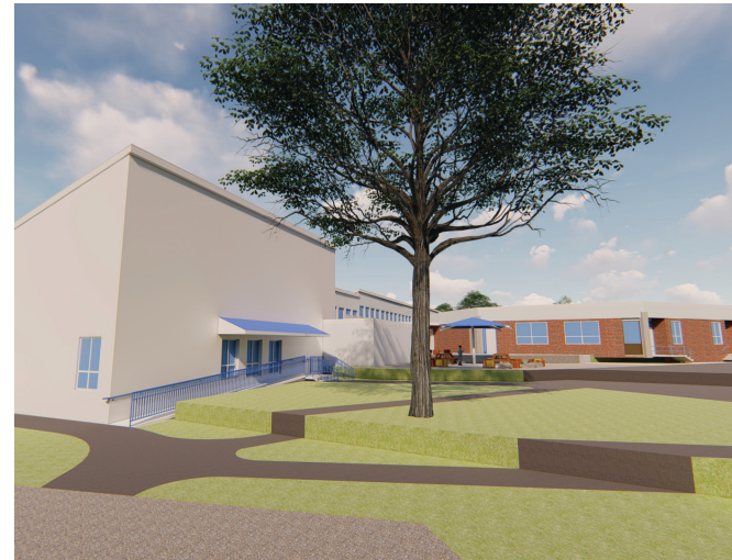
Media center from south
